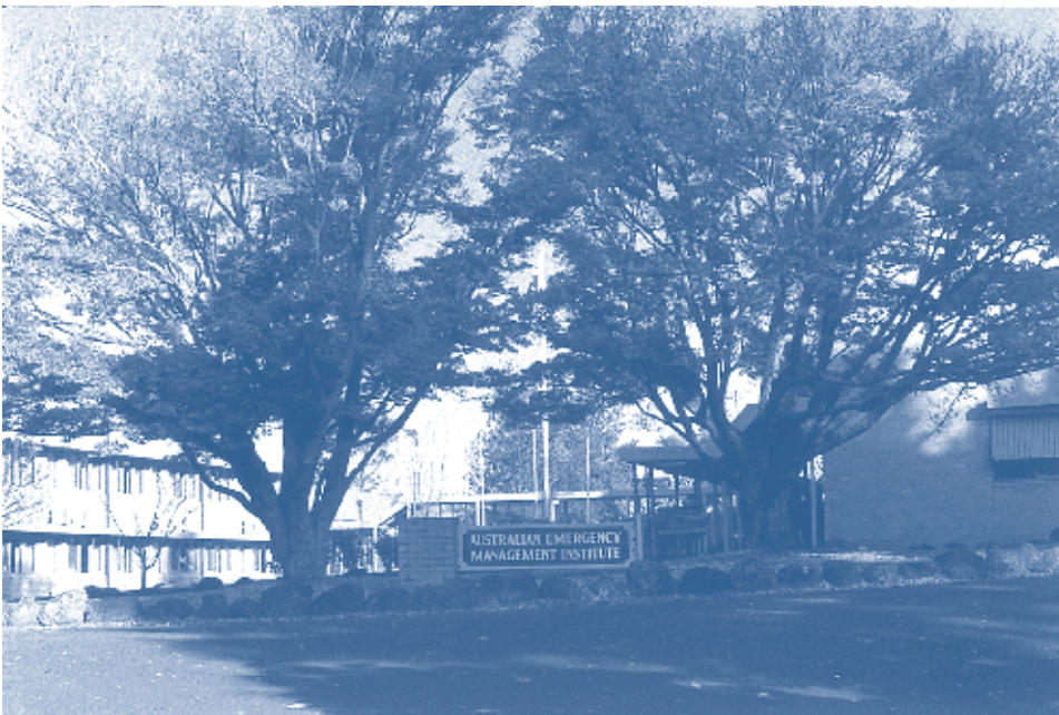
The Australian Emergency Management Institute located at Mt Macedon in Victoria.
