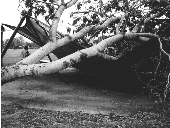
Typical shade sail damage from Cyclone Yasi in Townsville. TCC photo.
