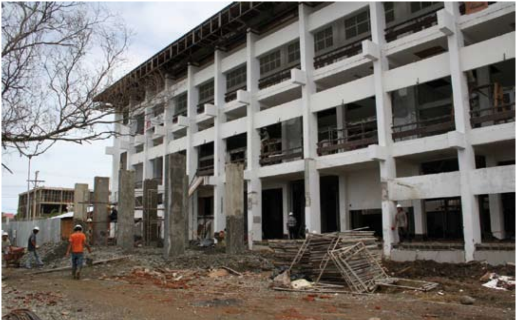
Construction at the emergency building, Zainoel Abidin Hospital, Banda Aceh.
