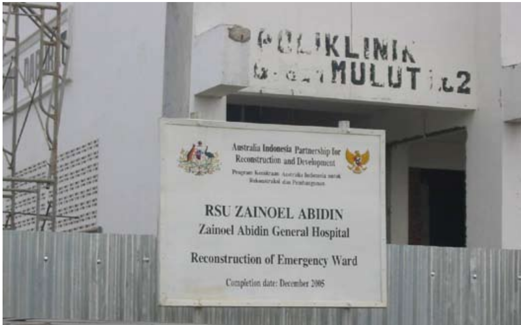
Construction works at the emergency ward building, Zainoel Abidin Hospital.
