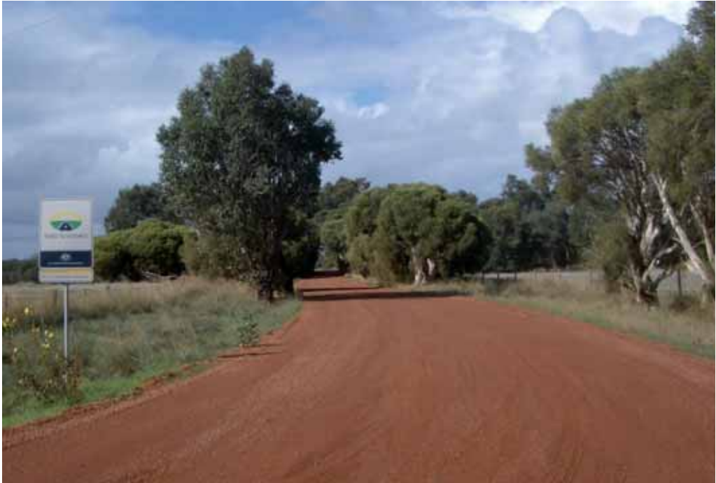
Shire of Serpentine Jarrahdale, Western Australia, Project No.25: Gravel road reconstruction, various sections of selected roads: strengthen formation and improve drainage ($69,042). Photo taken 12 May 2005.
