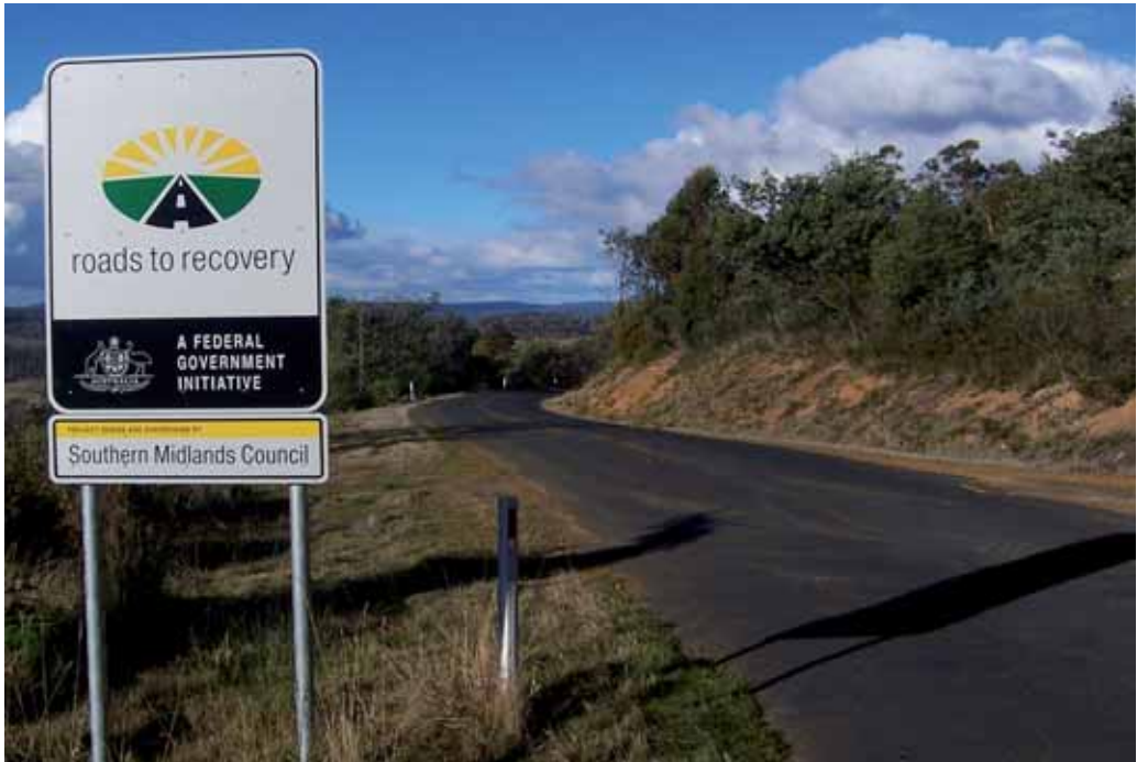
Southern Midlands Council, Tasmania, Project No.5: Woodsdale Road, Woodsdale: construct and seal present unsealed road including road widening and drainage. ($932,619 R2R cost with Council contributing the remainder of the estimated $2.1 million cost). Photo taken 7 July 2005.
