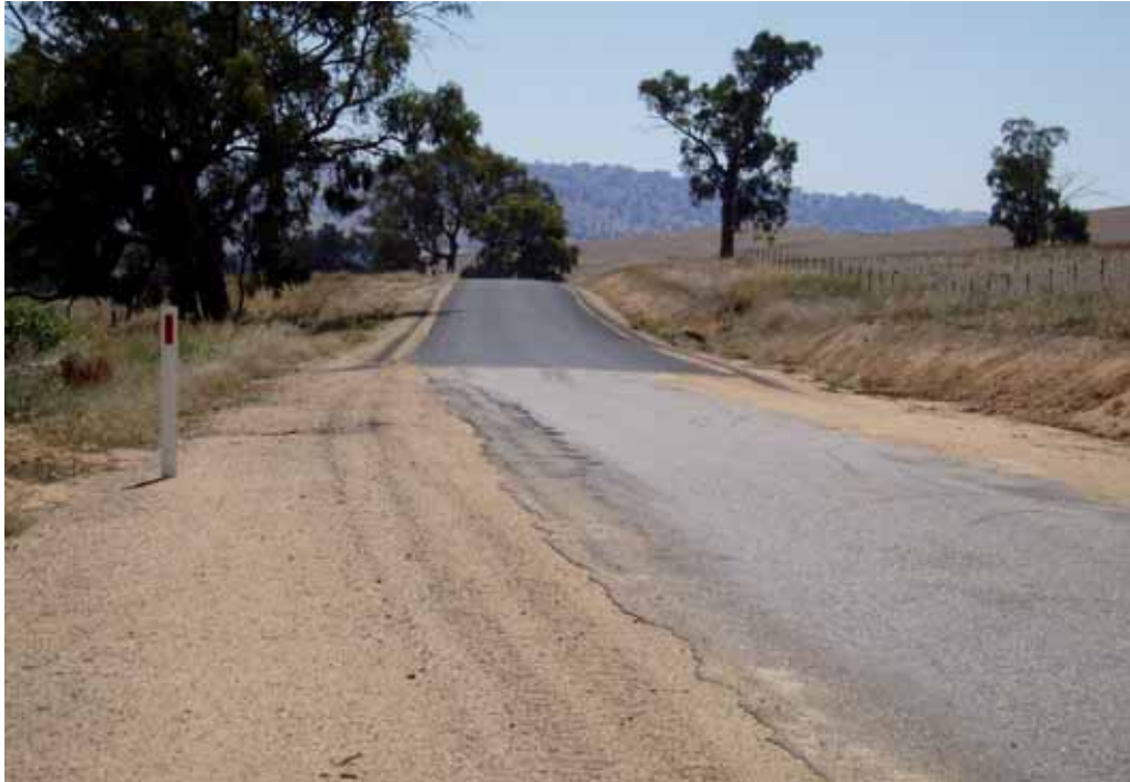
Gundagai Shire Council, New South Wales, Project No's 2, 6 and 8: Adjungbilly Road: widening carriageway and strengthening pavement ($263,204). Photo taken 14 March 2005.
