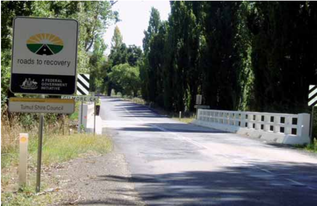
Tumut Shire Council, New South Wales: Project No.1: Main Road 279 (Gocup Road) from Chainage 1.2km to 2.9km—Excessive horizontal/vertical curves/alignments, inadequate lane widths and poor pavement strength. Realign, reconstruct, widen ($801,781). Photo taken 14 March 2005.
